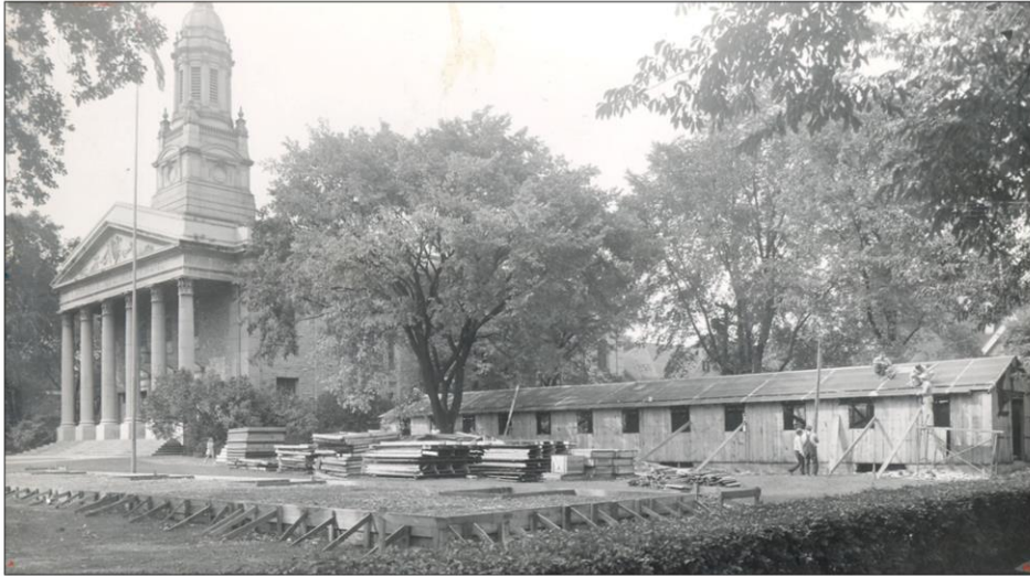
Barracks under construction next to the Chapel, 1946
